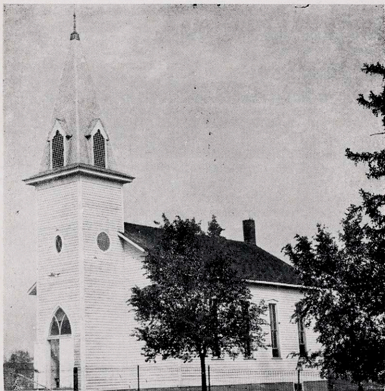
CENTER OF WORSHIP —This photo of Washington Reformed church, early house of worship for the Bilten settlement Swiss and others, might have been taken at the turn of the century. The sturdy building looks much the same today as it did when dedicated in 1876. The structure is believed to have been started in 1871 but the church records show the dedication was 73 years ago. (Times staff photo).
